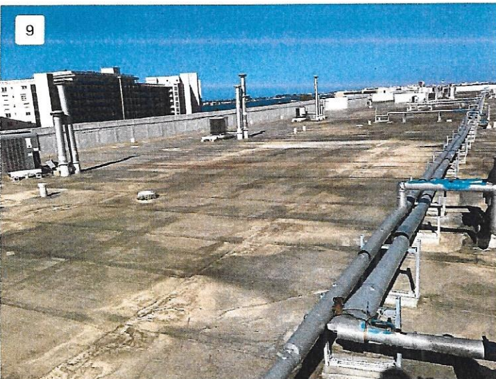
Overall of roof deck.
