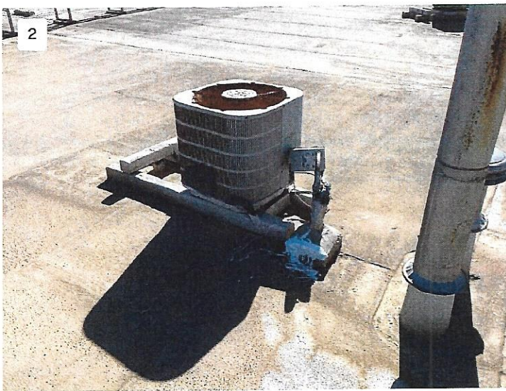
AC unit on sleepers directly on roof deck
