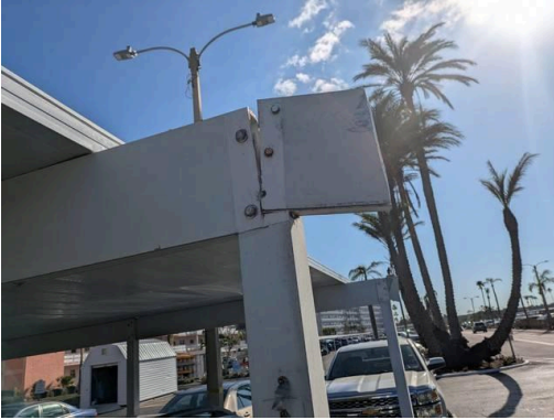
9 Damaged Structural Support
