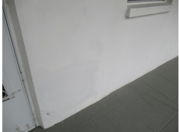
Previous stucco wall repair
