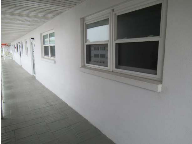
Typical stucco wall at breezeways
