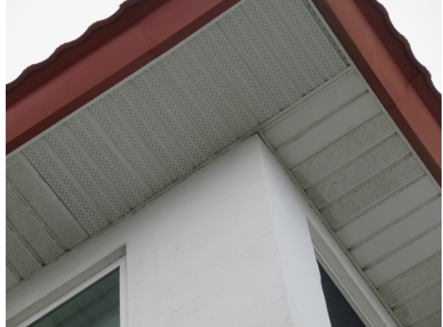
Soffit and fascia
