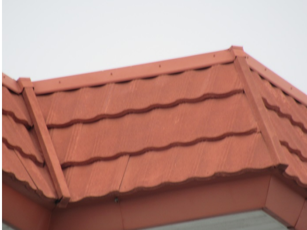
Typical metal mansard roof
