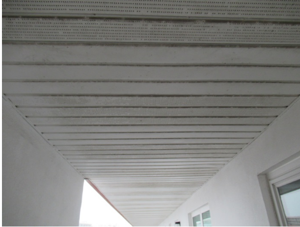
Soffit at breezeway
