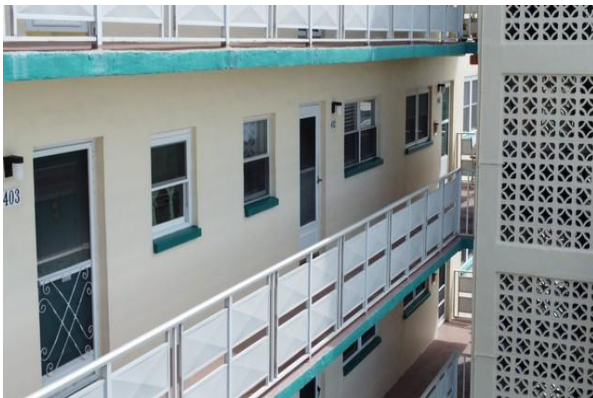
5 Walkway Railings Overview
