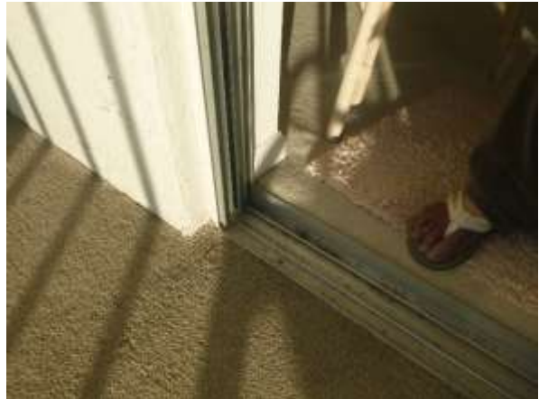
Photo 16: Track of Existing Sliding Glass Door
