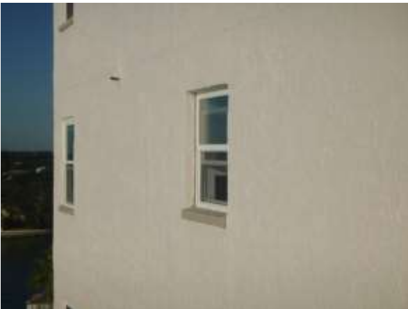
Photo 11: Exterior of Kitchen Window
