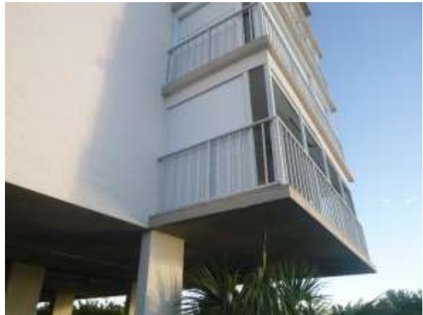
Photo 18: Exterior Wall at Unit 112
