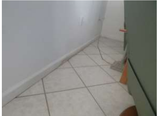
Photo 14: Wall at Unit 112
