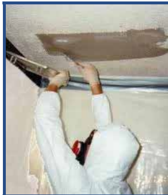
Licensed asbestos abatement worker removing asbestos-containing ceiling
