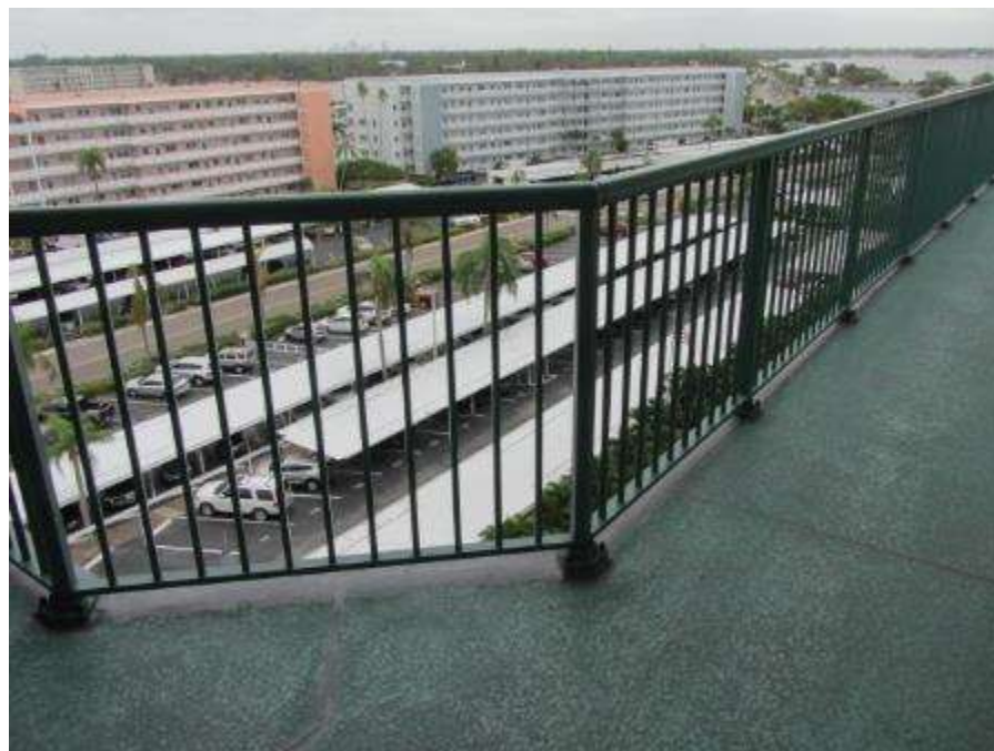
Photo #6 – Overview of guardrails and walkway looking from west to east.
