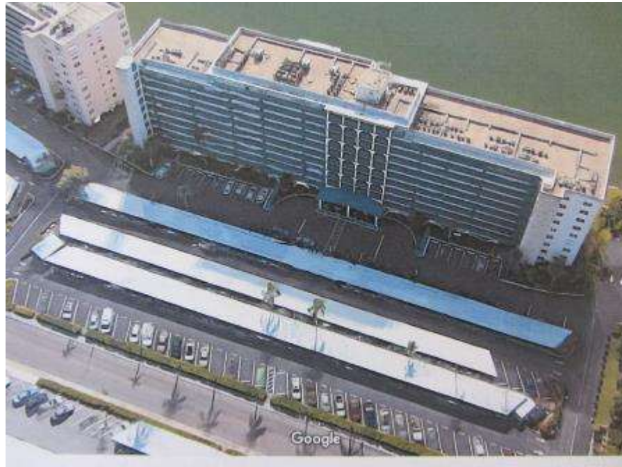
Photo #1 – Overview of front elevation
