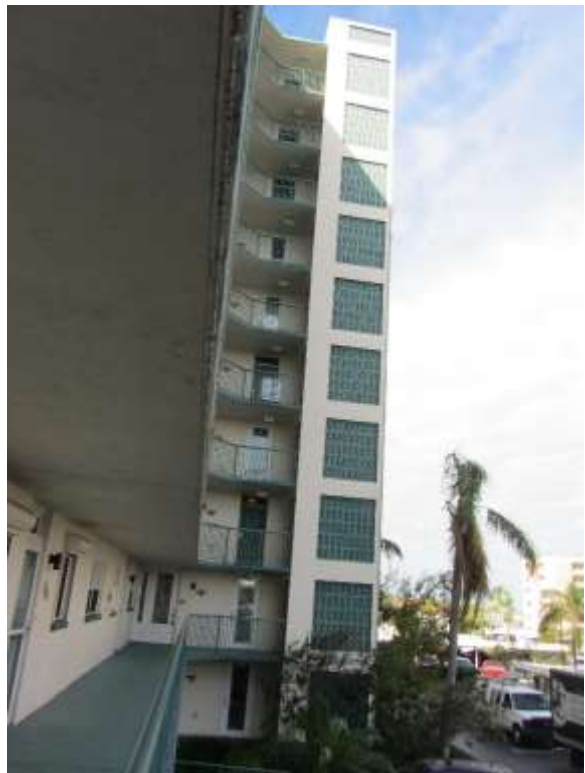
Photo #14 – West end stair tower
