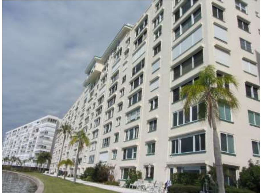
Photo #13 – Overview of rear (south) elevation of building
