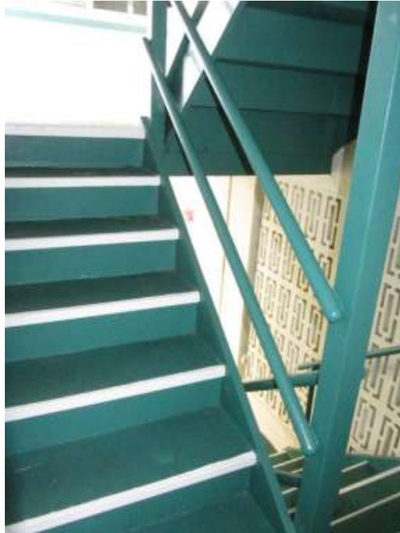
Photo #9 – Typical existing guardrail/handrail system in stair towers
