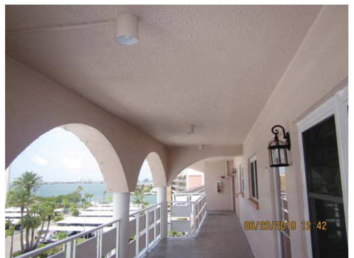
concrete deck attached to masonry wall
