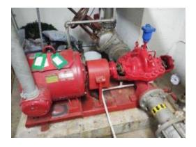
The fire pump was rebuilt in 2016 extending its life 30 years. The original age of the fire pump is 1981.
