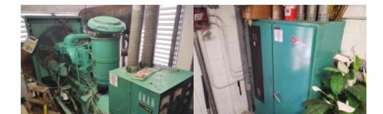
Photo is of the old generator and controller. This generator and controller were replaced in 2021 after completion of the reserve study.
