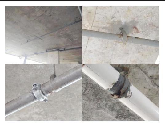
At the time of inspection partial repairs had been made to the fire sprinkler piping in the garage. A total of \$10,523.50 was spent in 2021 on partial replacements of piping and pipe hangers. The reserve allows for the replacement of the remaining fire sprinkler piping as well as pipe hangers located in the garage.
