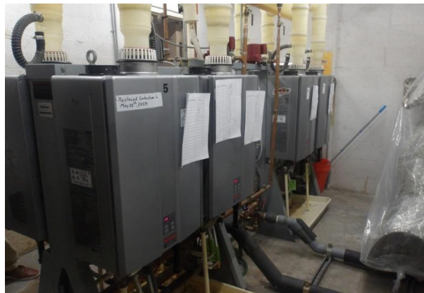
38 Buildings Tankless Water Heaters Overview
