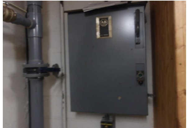
28 Domestic Water Pump Control Overview
