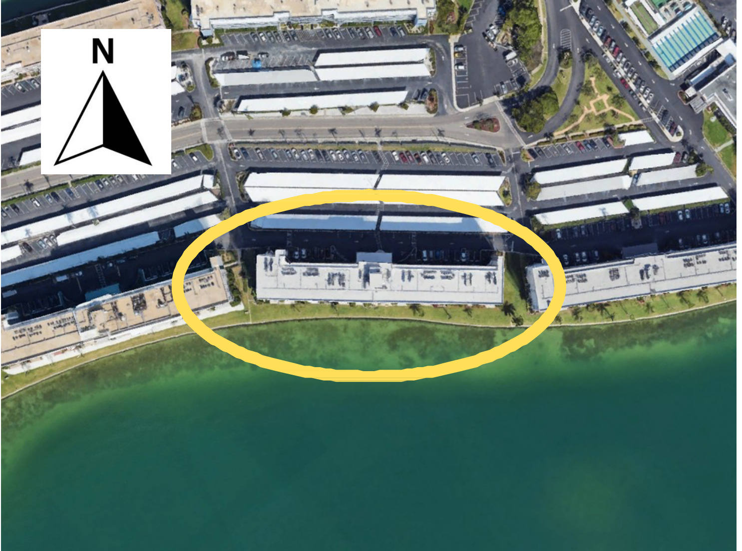
Plan view (overhead) image of the Diplomat House building at Town Shores of Gulfport.
