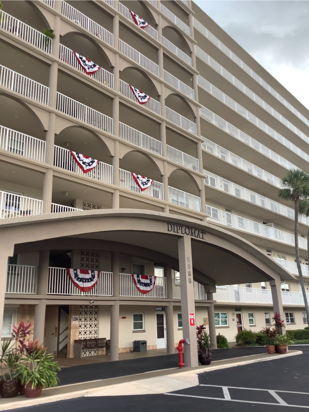
Exterior Elevation View (North)
