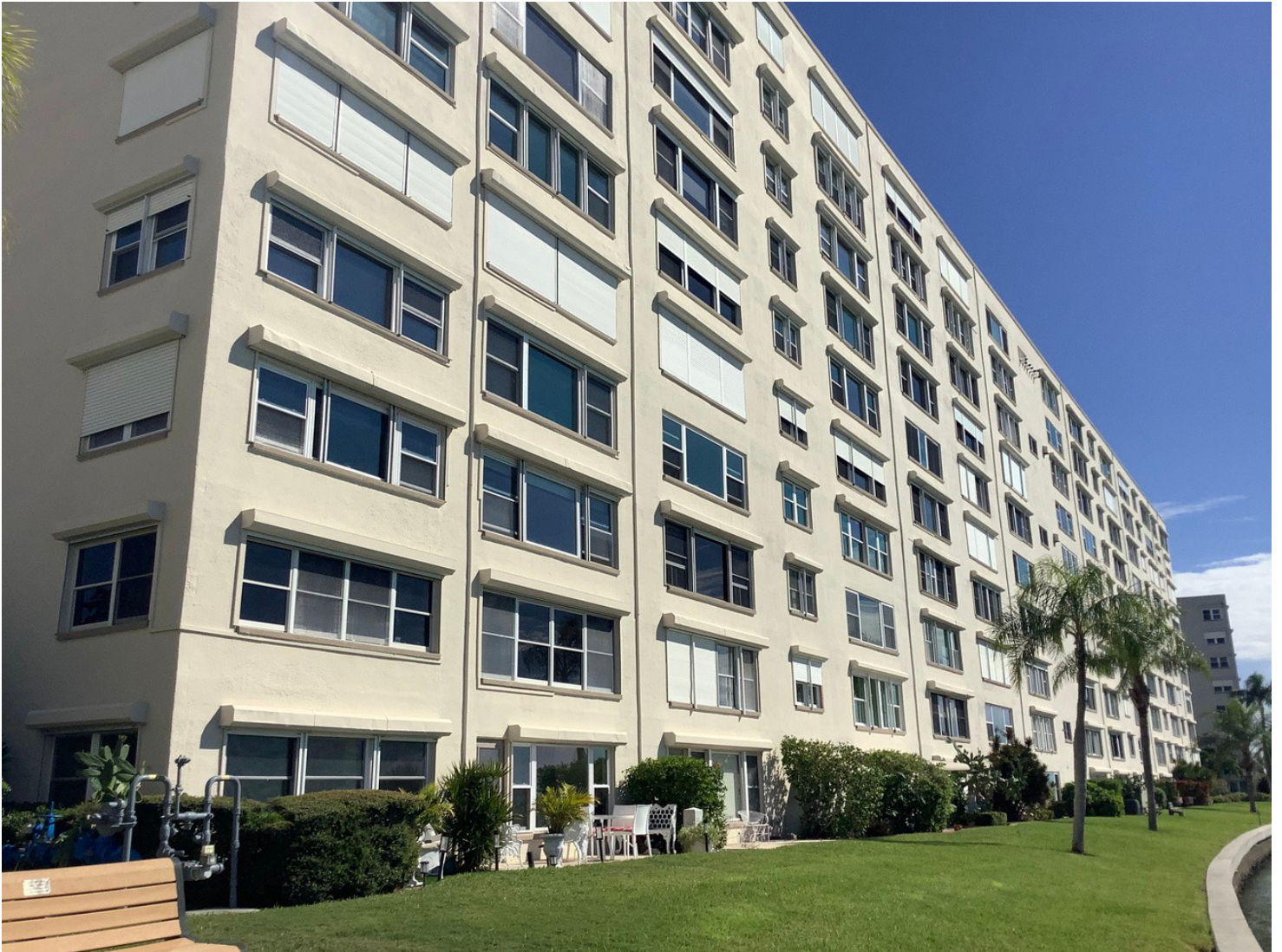
Exterior Elevation View (South)
