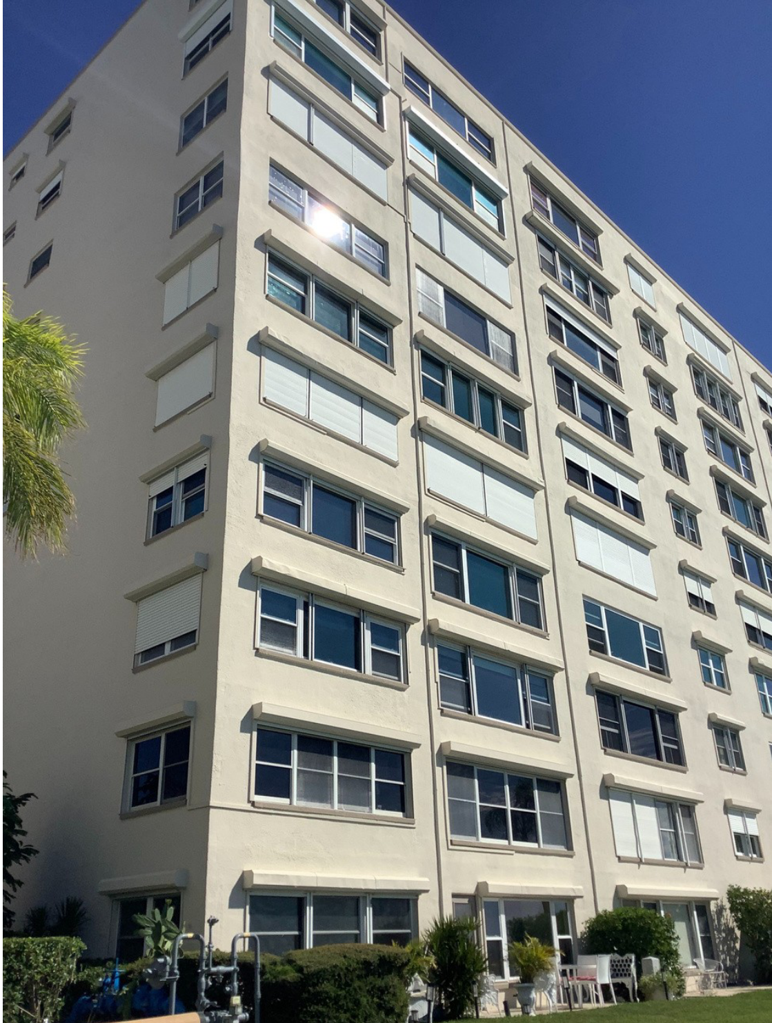
Exterior Elevation View ( West)
